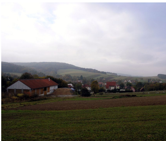
Figure 15: Biomass power plant in Hostětín (photo: WWF)
