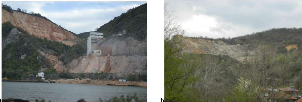
Fig. 14 Exploitation of construction materials (a) in the Djerdap National Park; open pit exploitation at Gura Văii (Iron Gates Natural Park)
