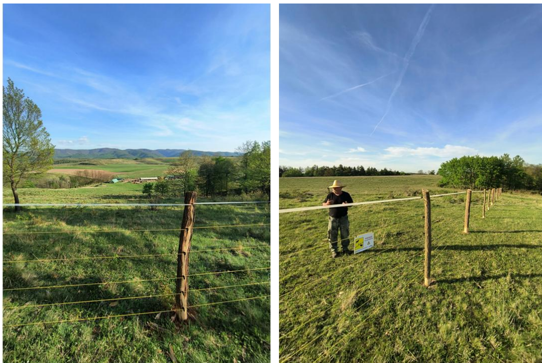
10. Figure - Multi-wire electric fence system installed in Nekézseny, within the Slovak-Karst & North Hungarian Mts. pilot area.
